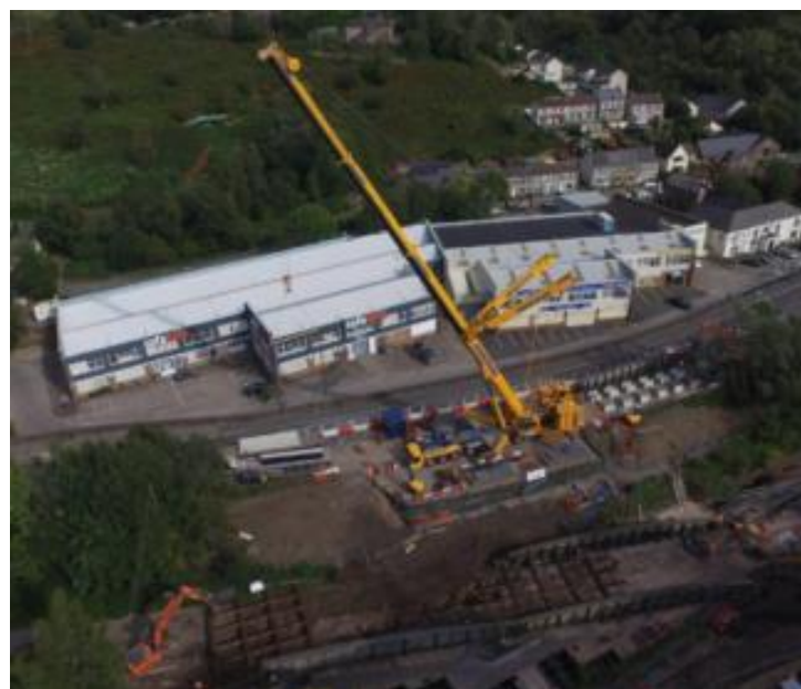
Plate 11. River Crumlin. 2021 Civils project of the year.
