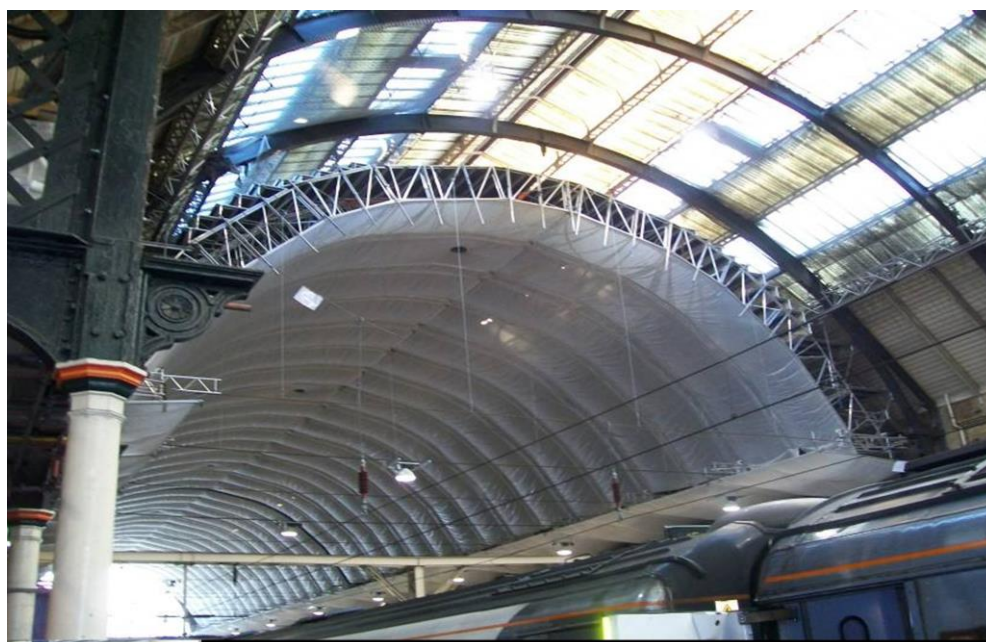
Plate19: Operational Station with Suspended Protection Deck.
