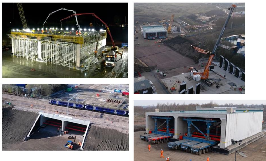
Plate 12. Ravenscraig Bridge SPMT move, 2023
