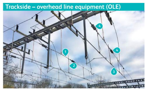
1. Catenary wire 2. Dropper 3. Contact wire 4. Insulators
