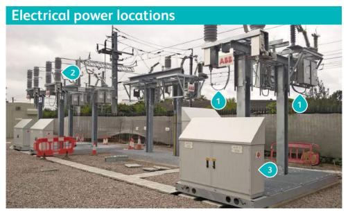
1. High voltage cables 2. Insulators 3. Switchgear cabinet
