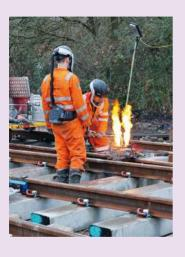
Hot work includes arc welding, thermit rail welds and rail grinding. Hazards are associated with the use of chemicals and gases, manual handling, high temperatures and hand arm vibration.
