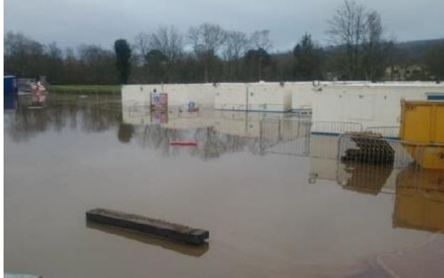
Polluted water contained within the site compound was now hazardous waste
