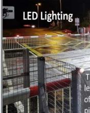
They produce a whiter light which improves the Closed-Circuit Television (CCTV) picture quality and provides better colour rendering. They also utilise multiple LEDs, which are not subject to degradation and lamp failure in the same manner as high pressure sodium and metal halide lamps.
