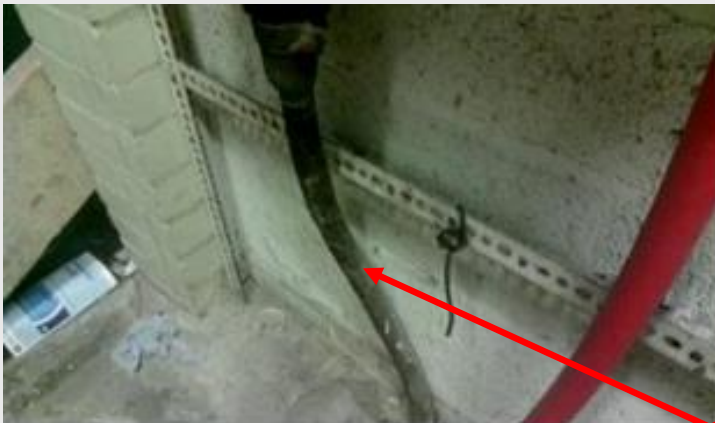
Wrap and bitumen coating
