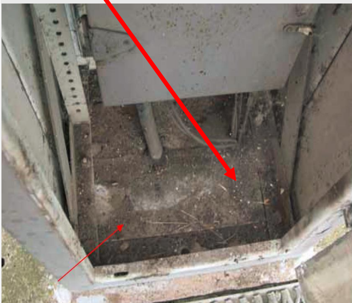
Asbestos Base Board
