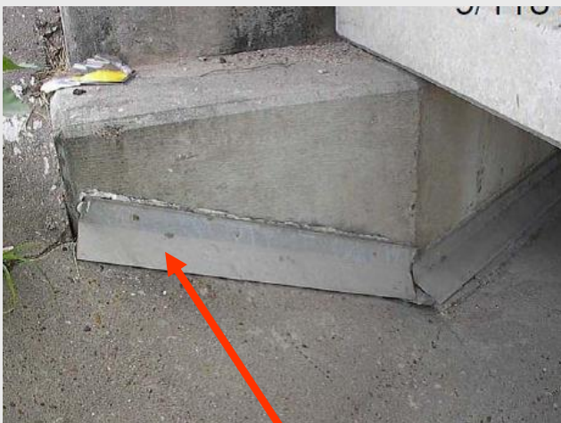
Mastic used to adhere flashing
