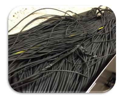
A mixture of working circuits & redundant wires as shown above is not uncommon.
