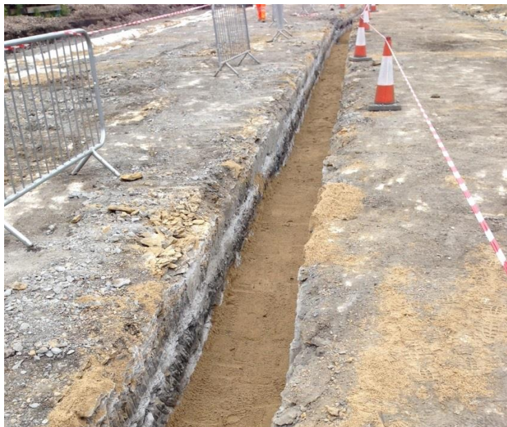
Photo 2 – Limestone trench excavated using a mechanical trencher
