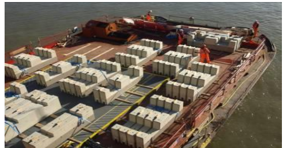
Prefabricated platforms being delivered by barge to Blackfriars
