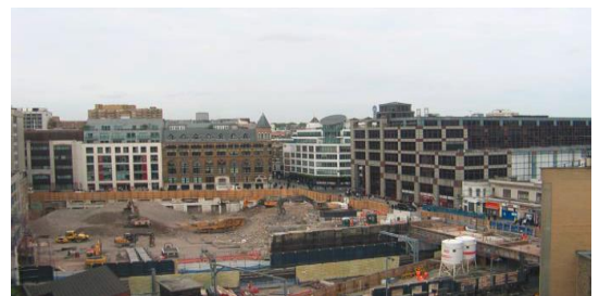
Use of demolition material as a piling mat at Farringdon
