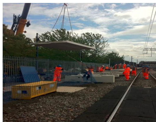
Prefabricated Platforms at Bedford Station
