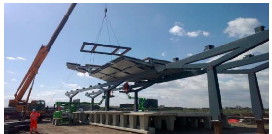
Prefabricated canopies at London Bridge Station
