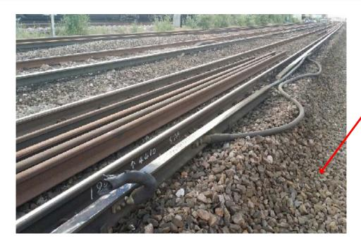
The investigation is underway and we know the cables were moved to allow the movement of tracked excavators along the ballast where a road had been removed
