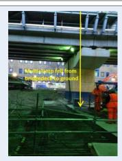
Platform 15 illustration of combisafe system with standard and clamp attached to concrete slab.
