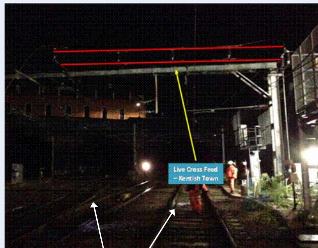
These roads were under possession and isolation
