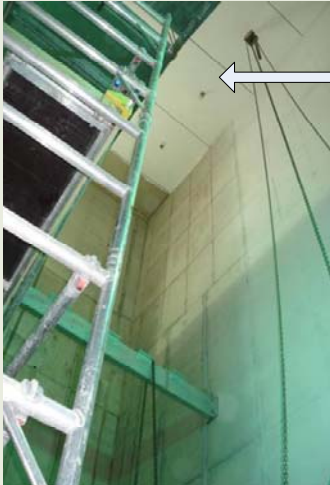
Socket where lifting eye was fixed
