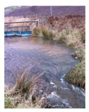
Failure to intercept and adequately redirect water from excavations before work starts.
