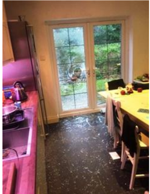
Damage to lineside neighbour's house
