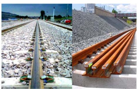
Well used rail provides a good conductive surface for track circuits, whilst rust on unused rails does not.
