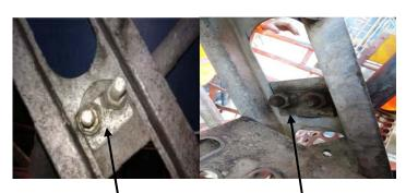
Inspection of the stair tower involved in the accident indicated that the locking plate had been fixed to the top of the 'stringer' resulting in the handrail fitting not being properly secured
