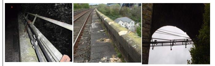
In May 2012 the handrail pulled out of the parapet and fell almost to ground level (photos above: centre and right): cable troughing fell to the road below and the parapet edge became inadequately protected to trackside personnel.
