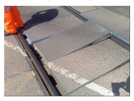
Note: The time taken from failure of the lug to the displacement of the panel appears to have been less than an hour. This is considered to be a new failure mode.
