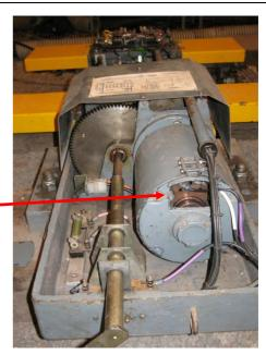
A small number of incidents have been experienced during routine maintenance work on the motor / drive mechanism of signalling points equipment caused by the ignition of flammable vapours.
