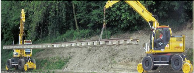
This picture is for illustrative purposes only - only scrap track panels are permitted to be lifted using unprotected chain slings.
