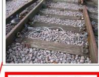
DO NOT 'LAY' THE SCS OUT ACROSS THE 4FT OR UNDER/NEAR THE CONDUCTOR RAIL OR ATTEMPT TO ATTACH THE CLAMPS TO ANY RAIL BEFORE THE ISOLATION HAS BEEN CONFIRMED
