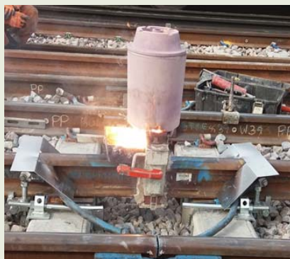
Alignment jig under trial
