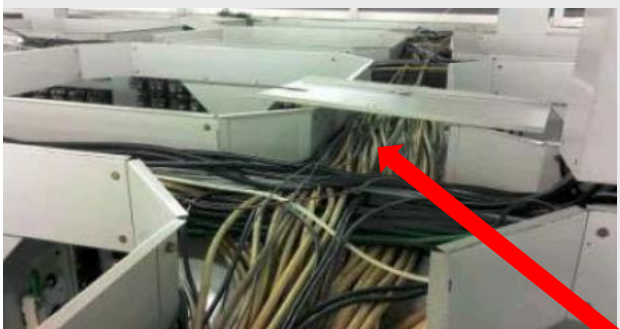
Debris within cable trays
