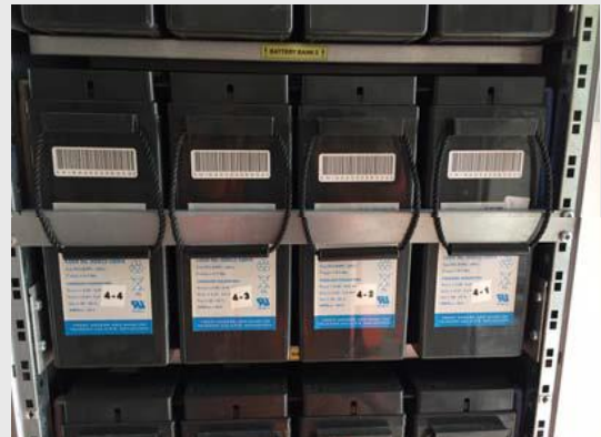
Battery String, Lead-Acid (Sealed)
