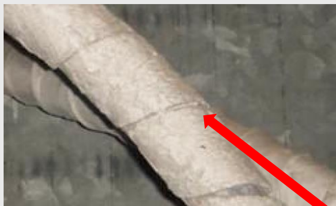
Paper insulation / cable sleeve
