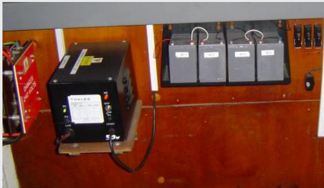
Battery Bank, Lead-Acid (Sealed)
