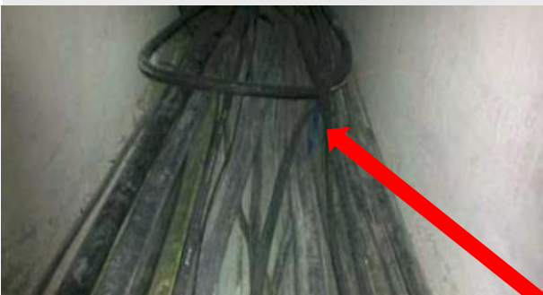
Debris within ducts
