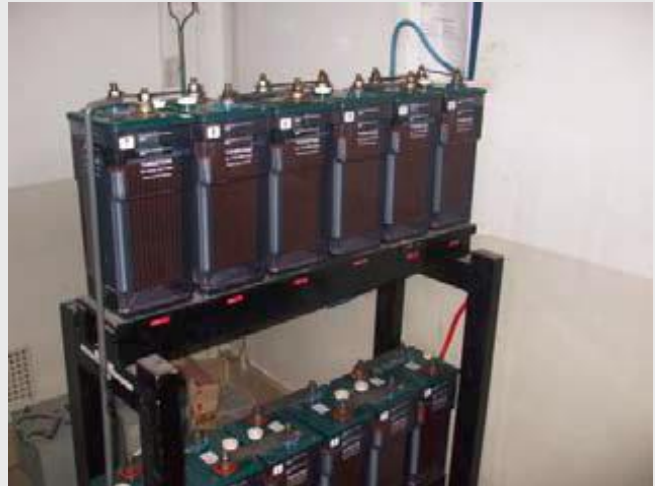
Battery Bank, Lead-Acid (Vented)
