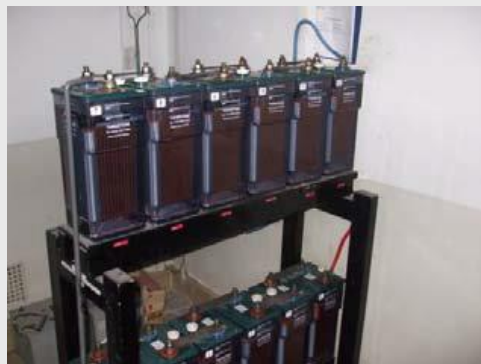
Battery String, Lead-Acid (Vented)
