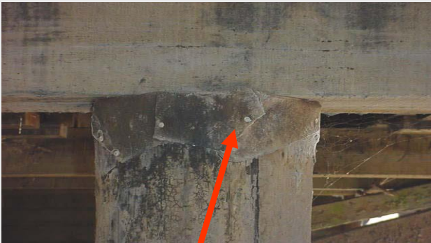
Roofing felt pile cap on timber bridge.
