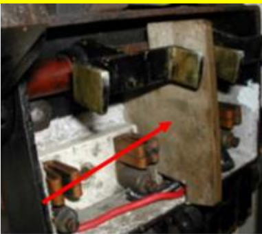
Fuse box/switch gear, fuse shields/flash guards – asbestos cement
