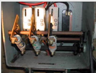
Fuse box/switch gear, fuse shields/flash guards – asbestos cement
