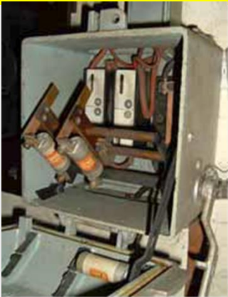
Fuse box/switch gear, fuse shields/flash guards – asbestos cement
