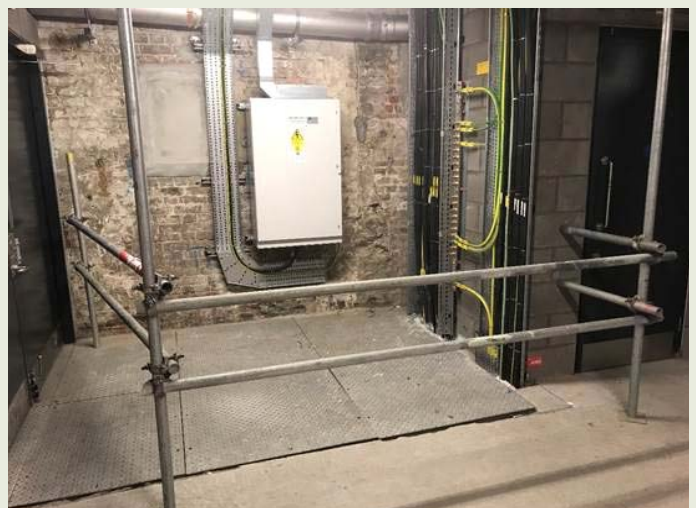
Scaffold handrail erected in the LV room.
