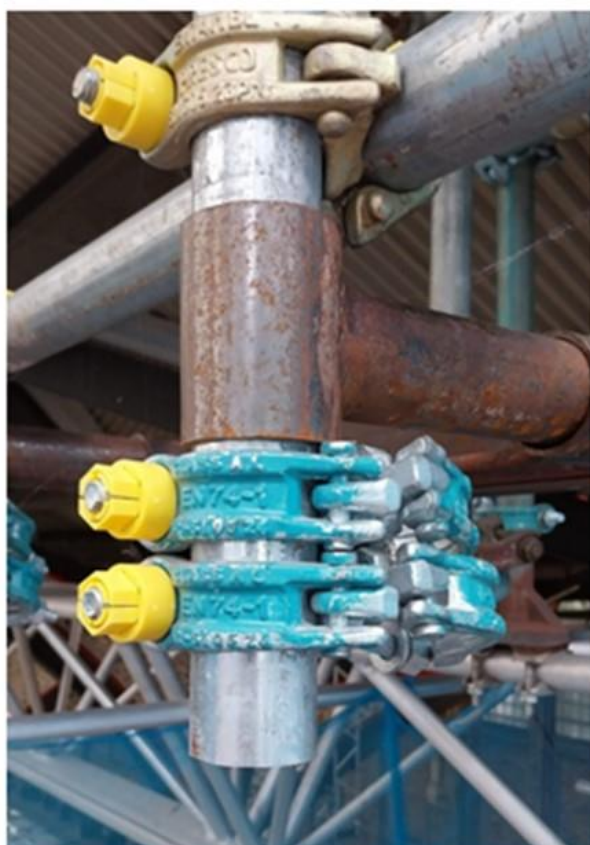
Revised detail with swivel coupler fittings permitting visual inspection of both fittings by erector. Note: Yellow Clikon caps to aid inspection.
