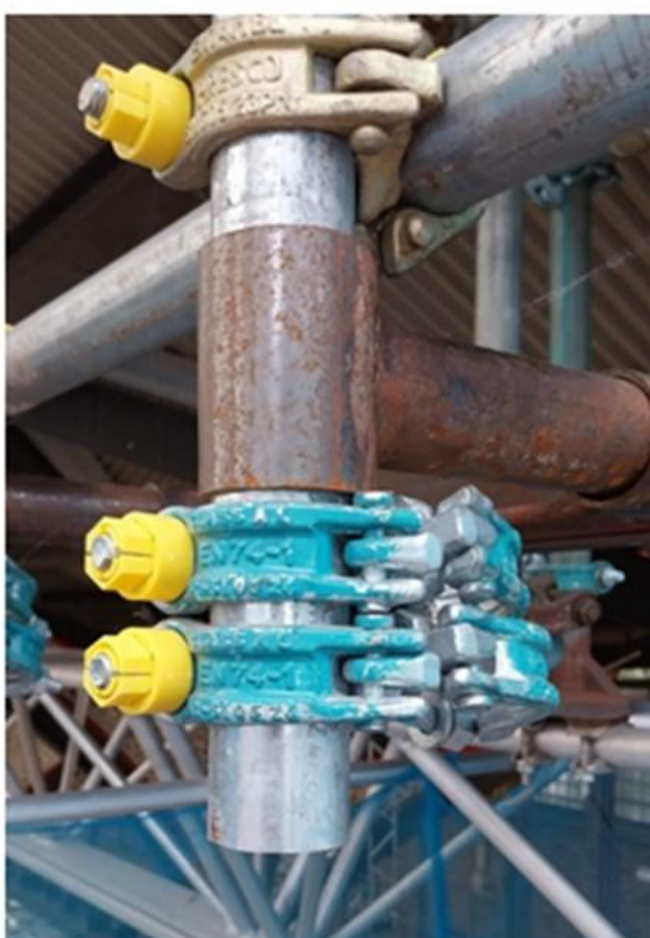
Revised detail with swivel coupler fittings permitting visual inspection of both fittings by erector. Note: Yellow Klikon caps to aid inspection.
