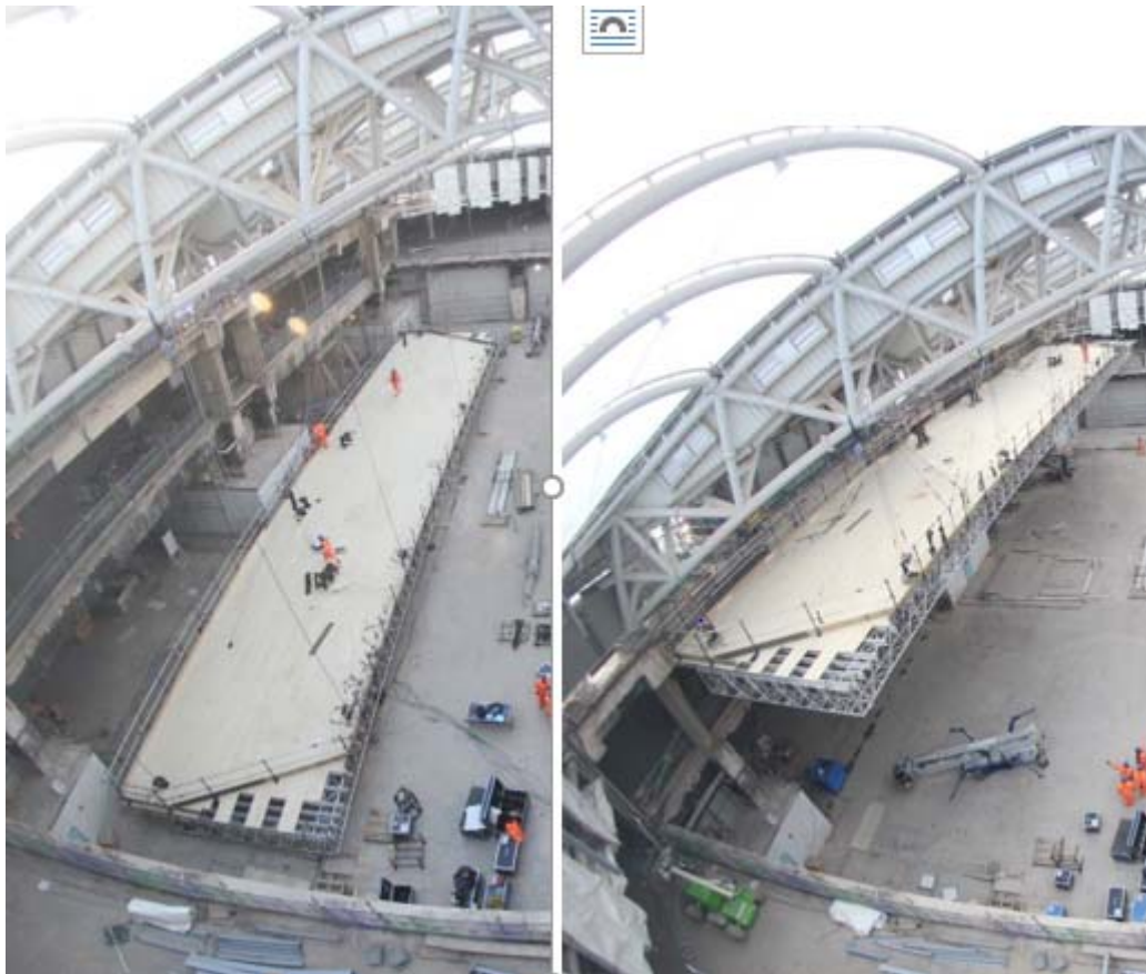
Plate 5: Birmingham New Street Atrium temporary decking.
