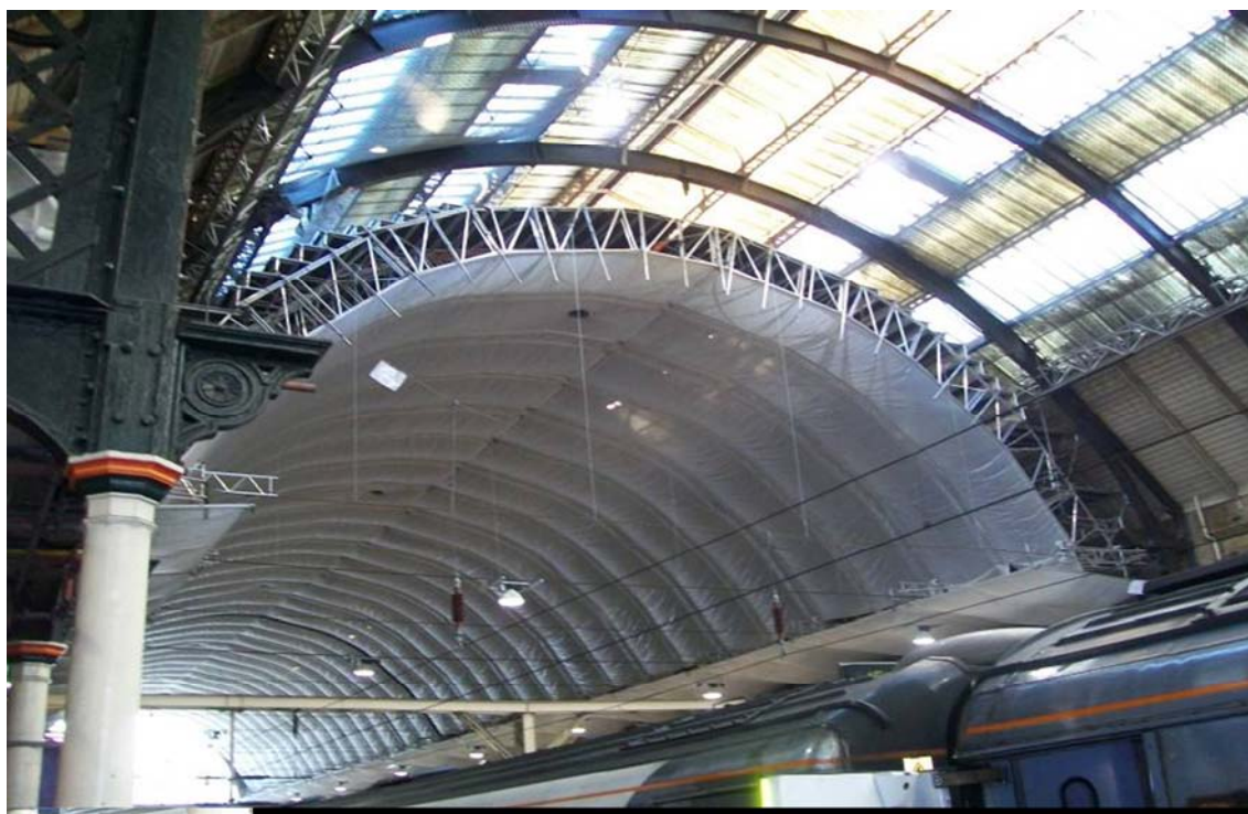
Plate 13: Operational Station with Suspended Protection Deck.
