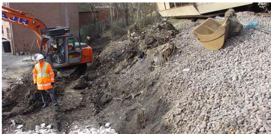
Plate 29: Temporary excavation to create works access road and site of derailed freight train at Cricklewood.
