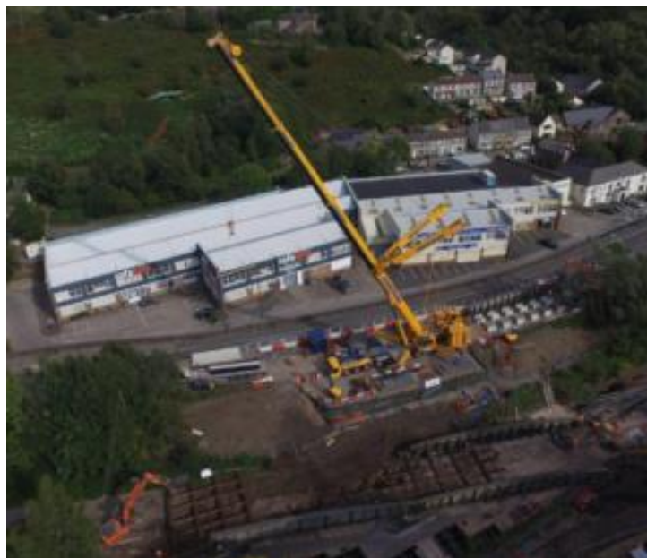
Plate 11. River Crumlin. 2021 Civils project of the year.
