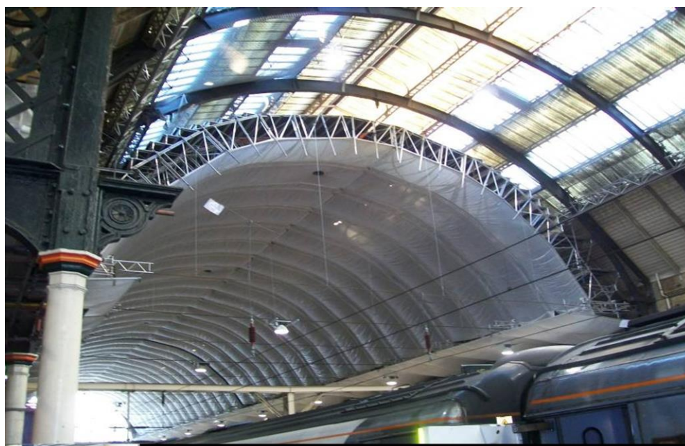
Plate 19: Operational Station with Suspended Protection Deck.
