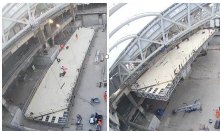
Plate 5: Birmingham New Street Atrium temporary decking.
