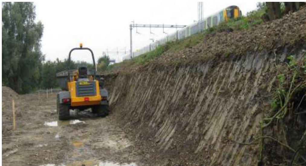
Plate 30: Bradwell Abbey toe cut contrary to (emerging) design, affecting track geometry (15 October 2013)
