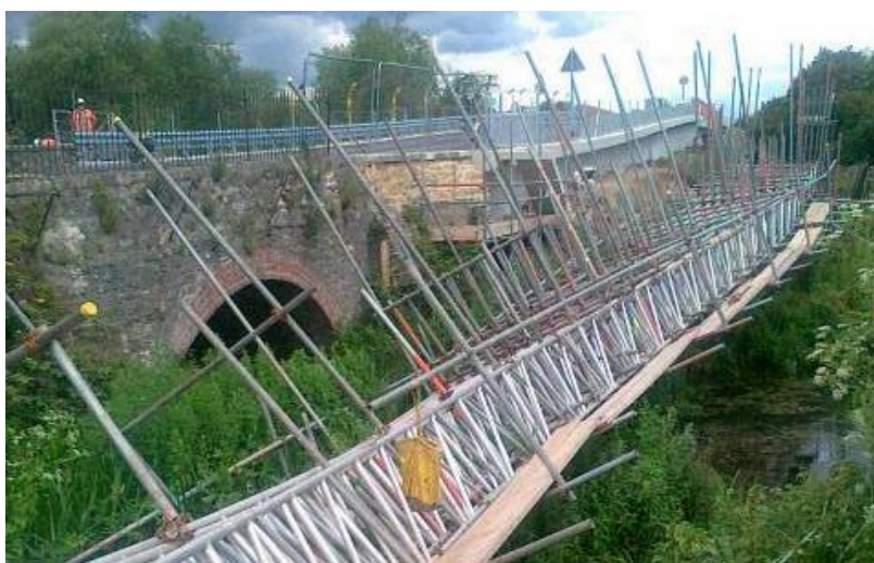
Plate 1: Collapsed Scaffold
