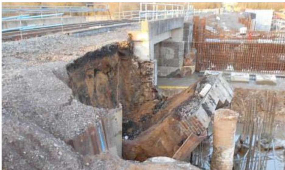
Plate 26: OXD39 Wingwall Failure due to undermining of existing structure during temporary works excavations.
