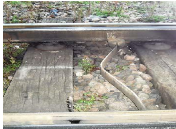
Stretcher Bar Damage
