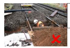
There is no Trench Support to prevent this individual being trapped if the sides of the excavation failed
