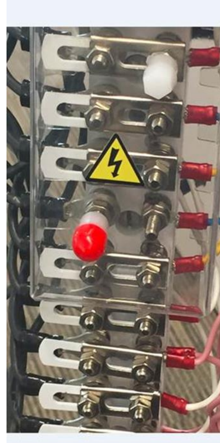
Shroud fitted to 2BA links
