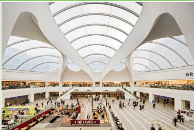
(Above) Birmingham New Street Station uses heat and electricity from a Combined Heat and Power (CHP) system, linked to a district heating scheme through Birmingham. The new CHP plant is located on the station roof and is much more efficient than conventional forms of heat and electricity provision.
