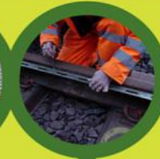
Cast and inspect the weld
