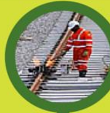
Cast and inspect the weld
