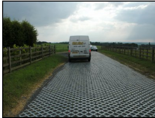
Typical Trackpave Installation along Access Track
