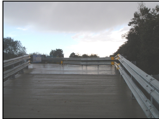
Armco Barrier – Bolted down to concrete surfacing
