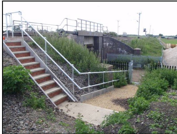
Brick & PCC flags – Pedestrian Access point
