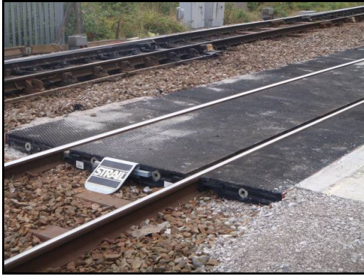
Proprietary Rubber Matting installed at RRV access point
