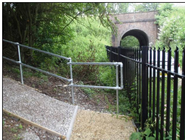
Pedestrian Ramp & Steel Handrail
