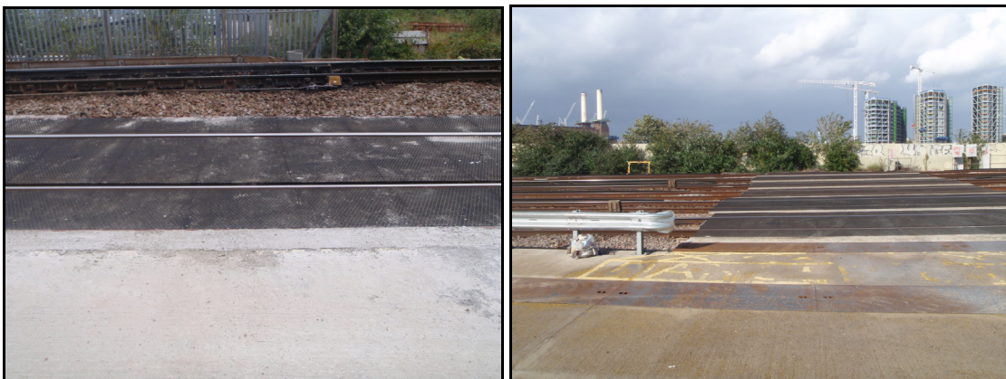
Concrete Apron installed at RRAP
