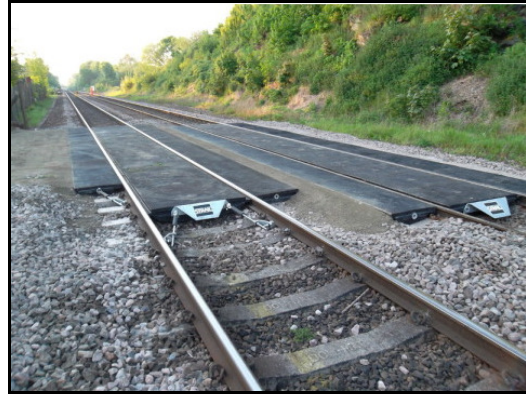
Proprietary Rubber Matting installed at RRV access point
