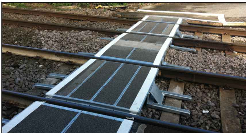
Polysafe system installed at pedestrian crossing point
