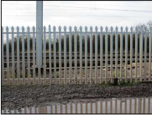
Palisade Fencing Installed along Railway Boundary
