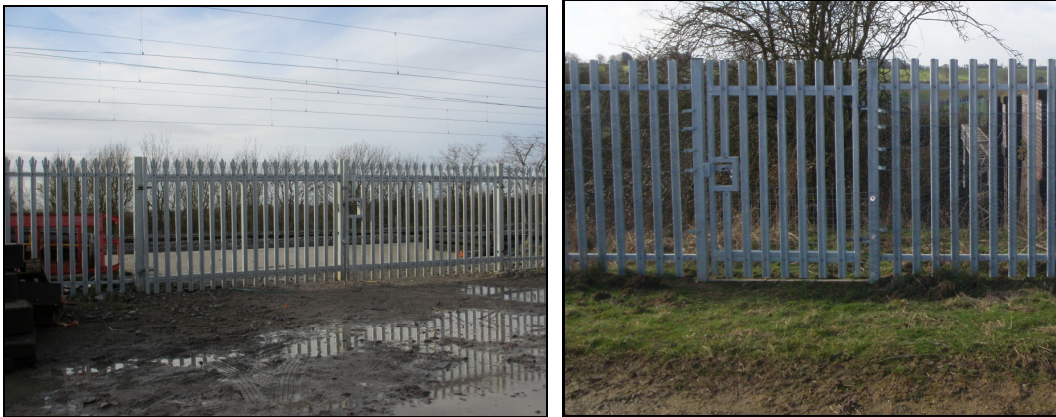
Palisade Vehicle & Pedestrian Access Gates
