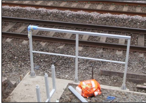
GRP/FRP handrail installed at the bottom of a steps
