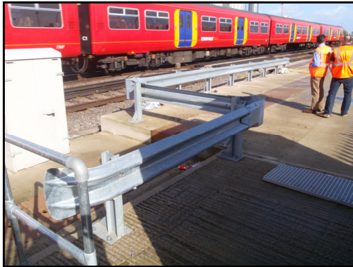
Armco Barrier – Bolted down to concrete surfacing
