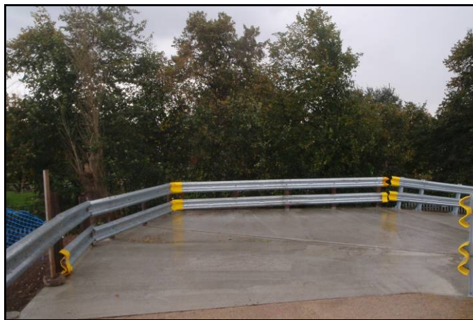
Concrete ramp up to track level
