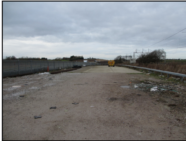
Rolled Stone Access Track within Network Rail Access Point
