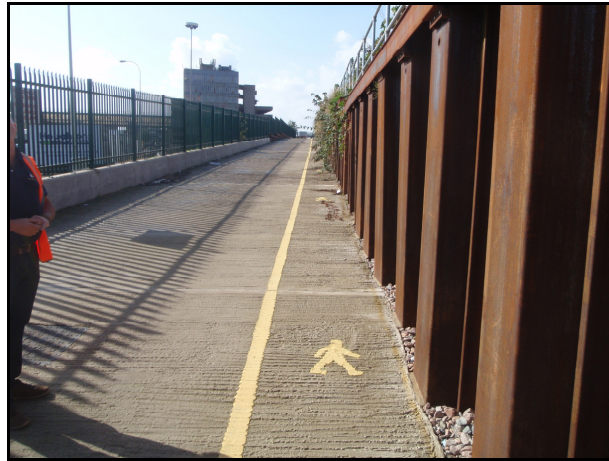
Designated pedestrian walkway to RRV access point
