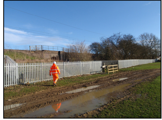
Palisade Fencing Installed along Railway Boundary
