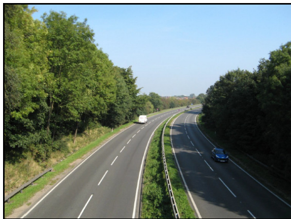
Asphalt Road / Surfacing
