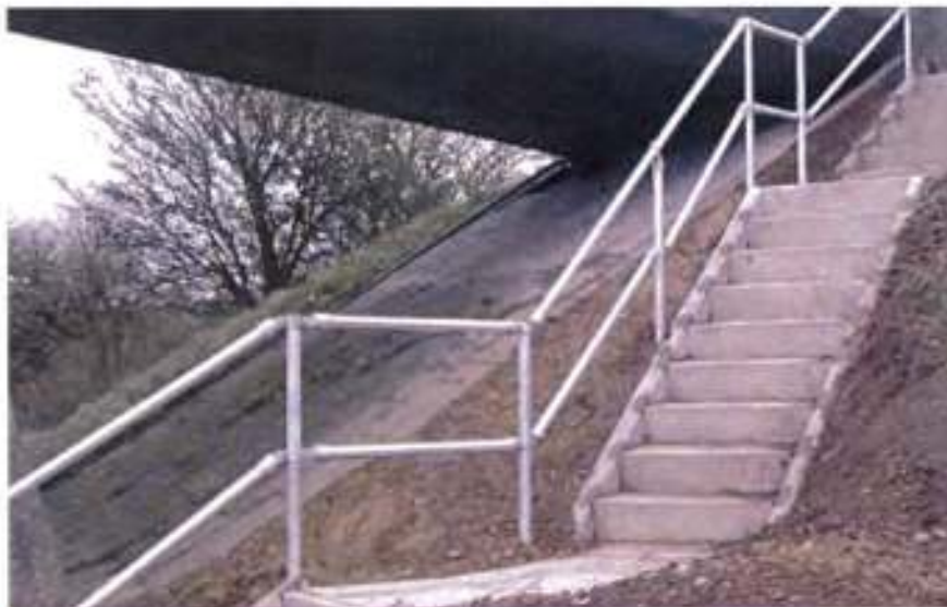
M4 embankment installation
