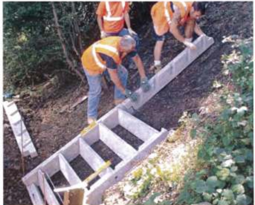
Modular components facilitate rapid installation
