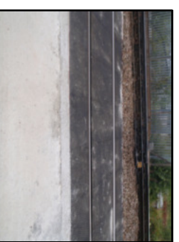
PHOTO A - MATTING AND CONCRETE APRON
