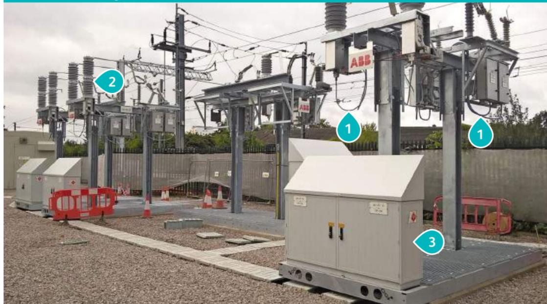
1. High voltage cables 2. Insulators 3. Switchgear cabinet
