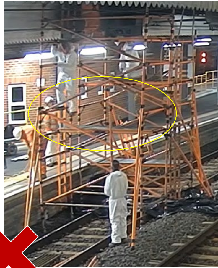
Missing platform under handrail section increasing size of fall if op was to slip from handrail section.
