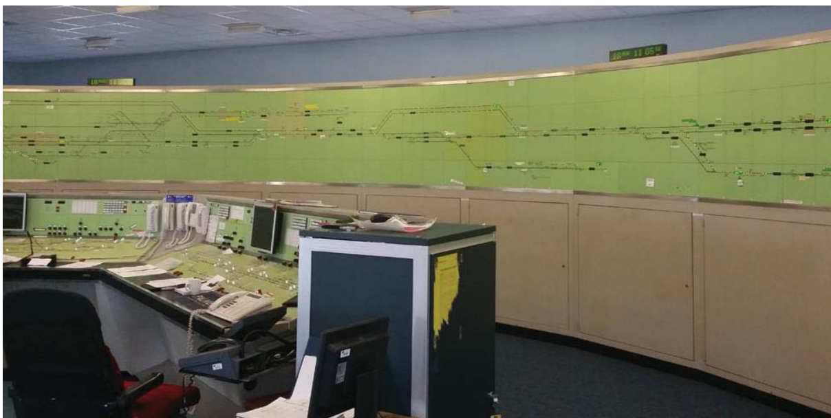
General view of Westbury signal box
