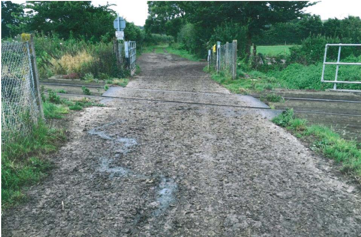
Thorney Marsh Lane level crossing (photo courtesy of Network Rail)
