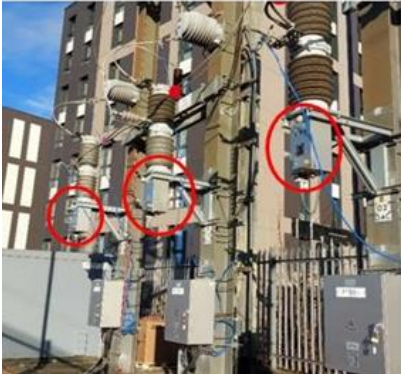
Rating plate in HV Pole, located at the magnetic actuator enclosure.
