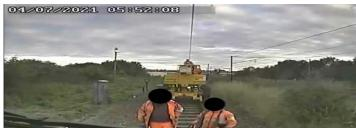
Machine Controller and Crane Controller walking in the four foot between the MEWP and RRV which is travelling in reverse back to Springfield RRAP
