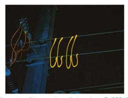
Illustration of incorrectly applied earths at E/306/05
