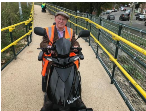
Dorchester accessibility ramp
