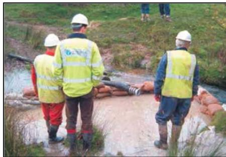
It is delivered to site as a powder or as granules before being mixed with water. The mud or slurry is pumped to where it is being used and then the excess is cleaned up.
