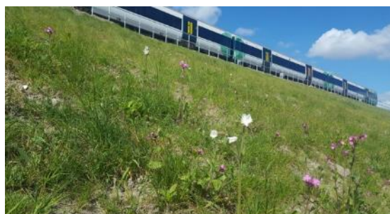
Fig. 26 Bermondsey Dive-Under wildlife embankment
