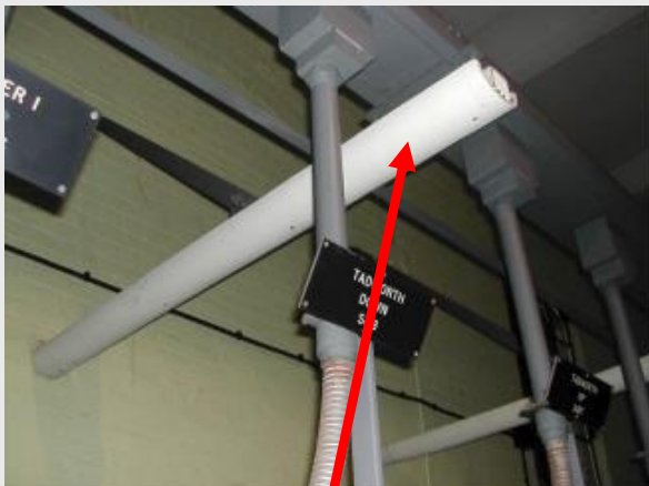
Above Circuit Breakers Cable Troughs (Cement)
