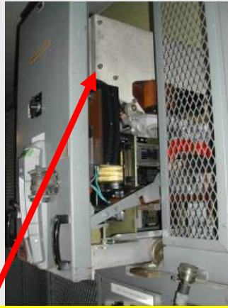
D.C. Circuit Breaker Arc Chute
