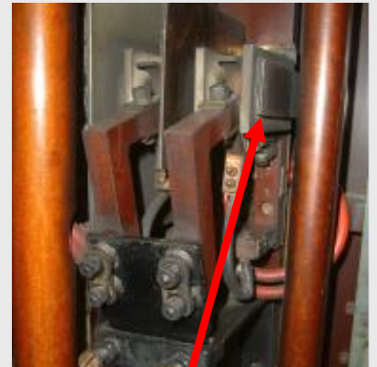
Circuit Breaker Main Isolator (Cement Flash Guards)
