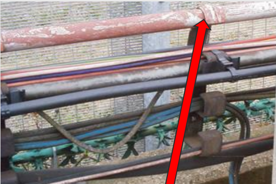
Packing to cable hangers
