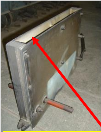
D.C. Circuit Breaker Arc Chute
