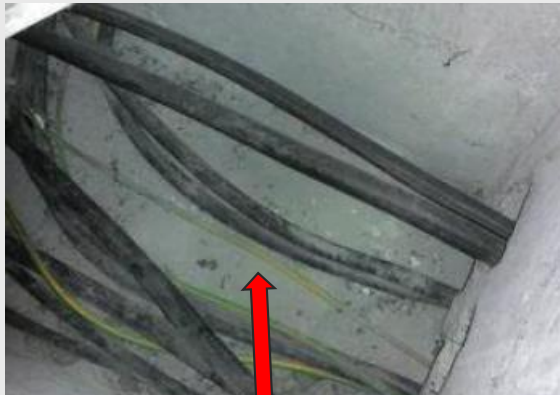
Cable run with dust/debris
