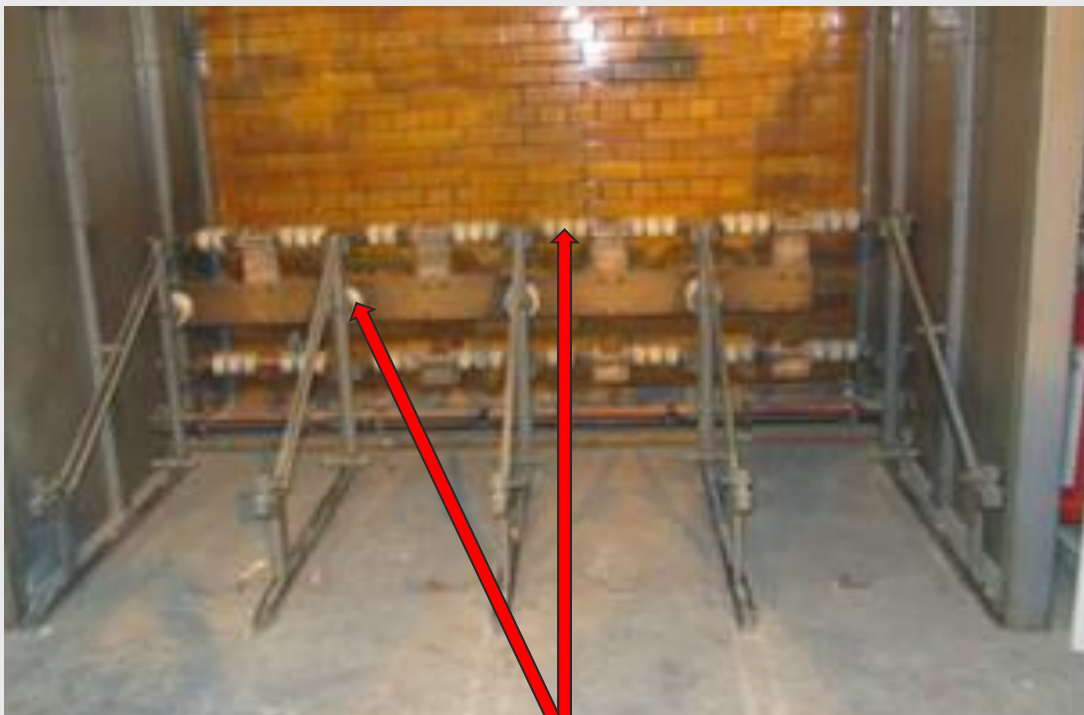
Packers / spacers (DC Busbars)
