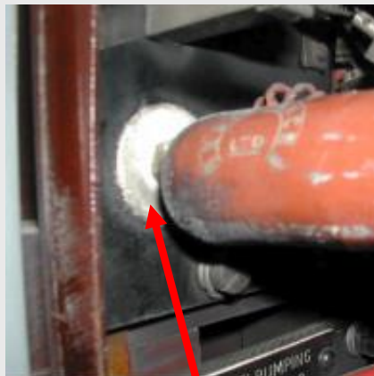
Circuit Breaker, Washer to Resistor
