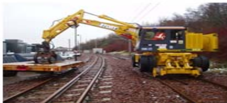
Road Rail Vehicle (RRV)
