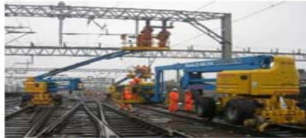
Mobile Elevated Work Platform (MEWP)
